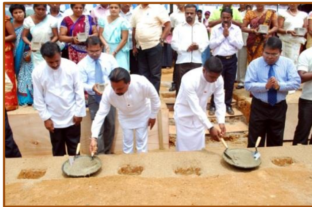
Laying foundation stone for the commencement of the project
